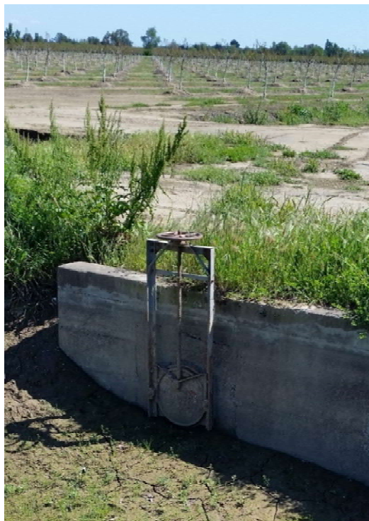
Figure 6-5 Canal Turnout Gate with Trash Rack
