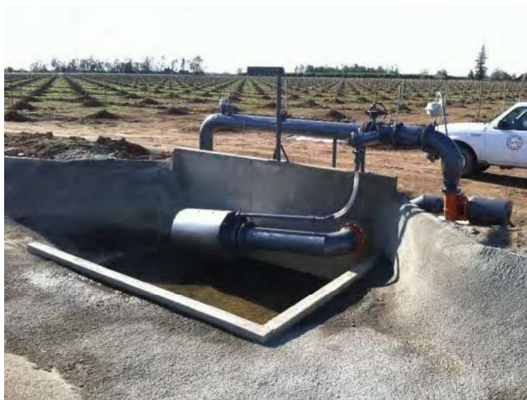
Figure 3. Alternative turnout structure to allow direct pumping from district canal to supply an on-farm pressurized irrigation system. During and following construction.
