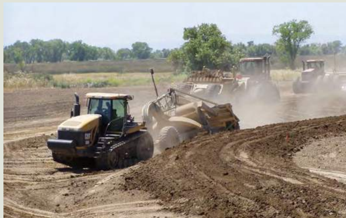
Levee construction for wetland habitat restoration, Gray Lodge Wildlife Area - Ducks Unlimited, Inc.
