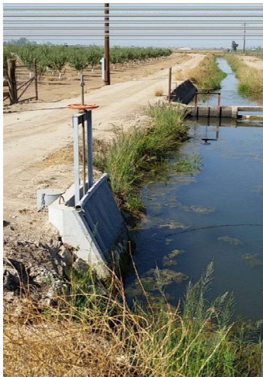
Figure 6-5 Canal Turnout Gate with Trash Rack
