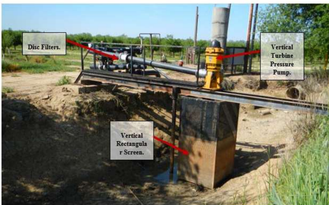
Figure 6-11 Vertical Rectangular Screen Protecting Vertical Turbine Pressure Pump, Followed by Disc Filters for Prune Irrigation with Microspray
